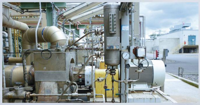
IDP pump with seal supply unit in application at TOTAL Leuna.
